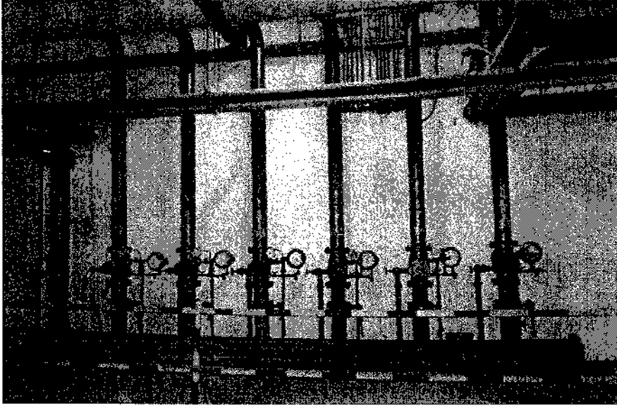
ACV FOR AUTOMATED SPRINKLER
