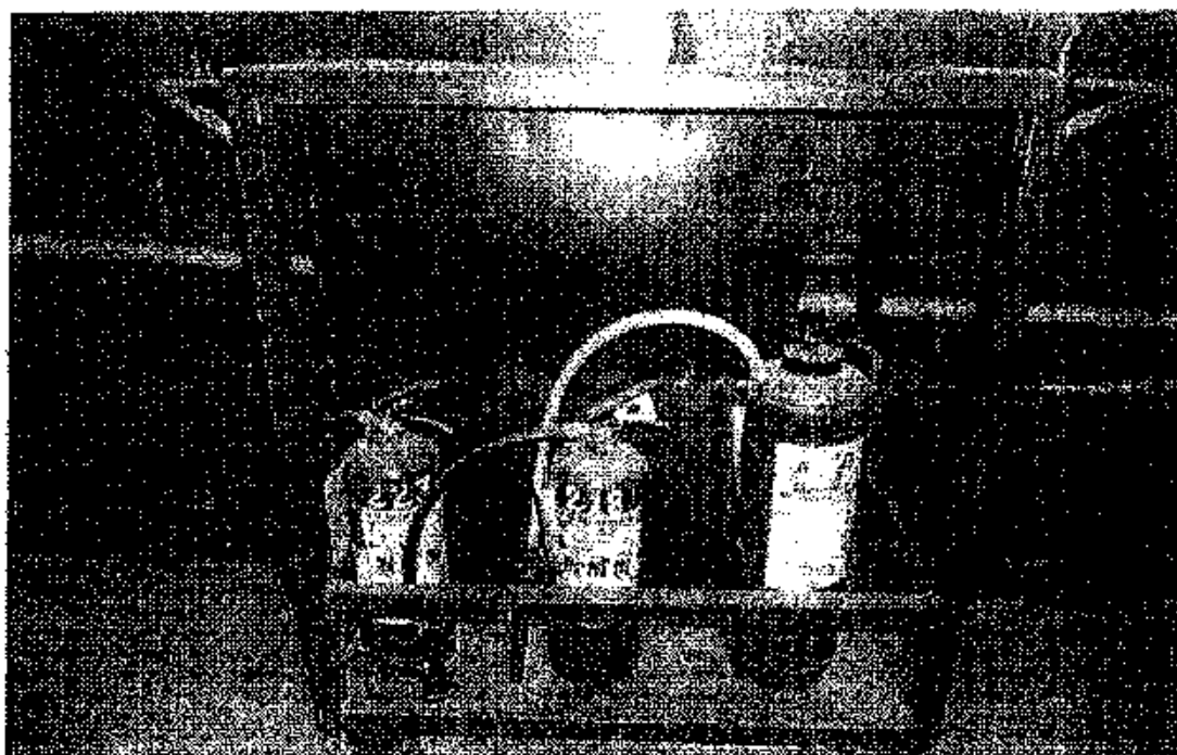
PORTABLE EXTINGUISHERS ON TROLLEY
